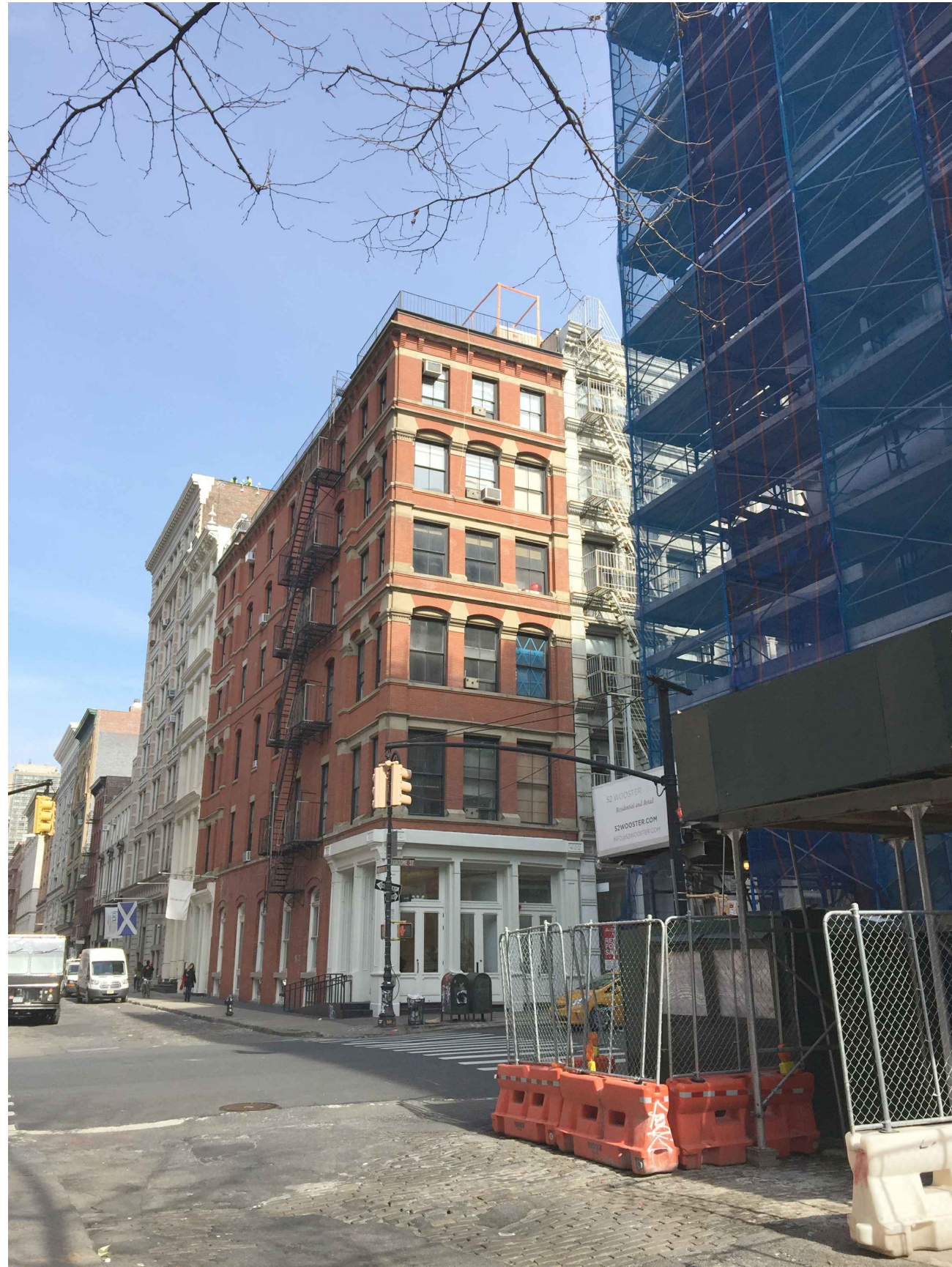
2 PHOTO OF MOCK UP OVER EXIST. BULKHEAD (VIEW FROM WOOSTER ST.)
